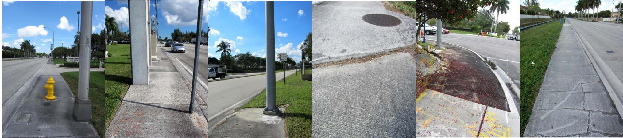
*Issues encountered during a Field Analysis included (From Left to Right): Non-ADA compliant sidewalks, infrastructure obstacle course, missing sidewalks, uneven sidewalks, post maintenance issues, cracked sidewalks*
